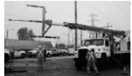
Once energized conductors are secured and moved out of the work zone using the remote controlled Robotic Arm, work can safely proceed to perform any maintenance that is required.
