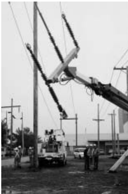
The Robotic Arm has the ability to adapt to all wire configurations and is available in four different weight capacities and sizes. It can be controlled from the ground or from an elevated position remotely while maintaining safe limits of approach while conductors are moved into the required position.
