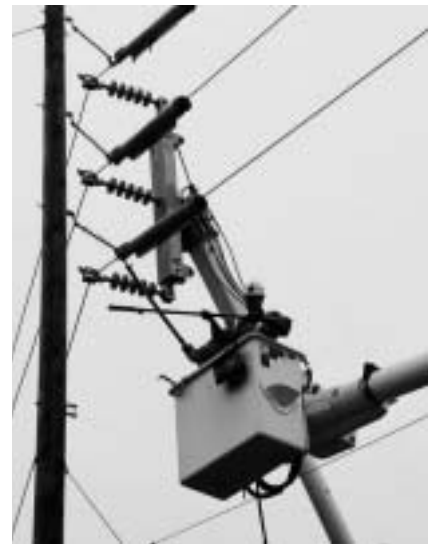
Once energized conductors are secured and moved out of the work zone using the remote controlled Robotic Arm, work can safely proceed to perform any maintenance that is required.
