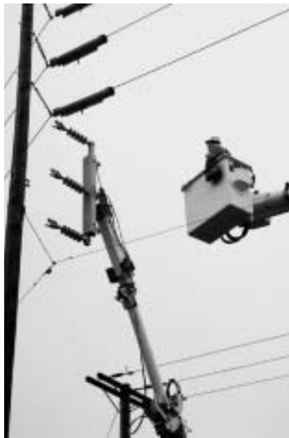
The Robotic Arm has the ability to adapt to all wire configurations and is available in four different weight capacities and sizes. It can be controlled from the ground or from an elevated position remotely while maintaining safe limits of approach while conductors are moved into the required position.
